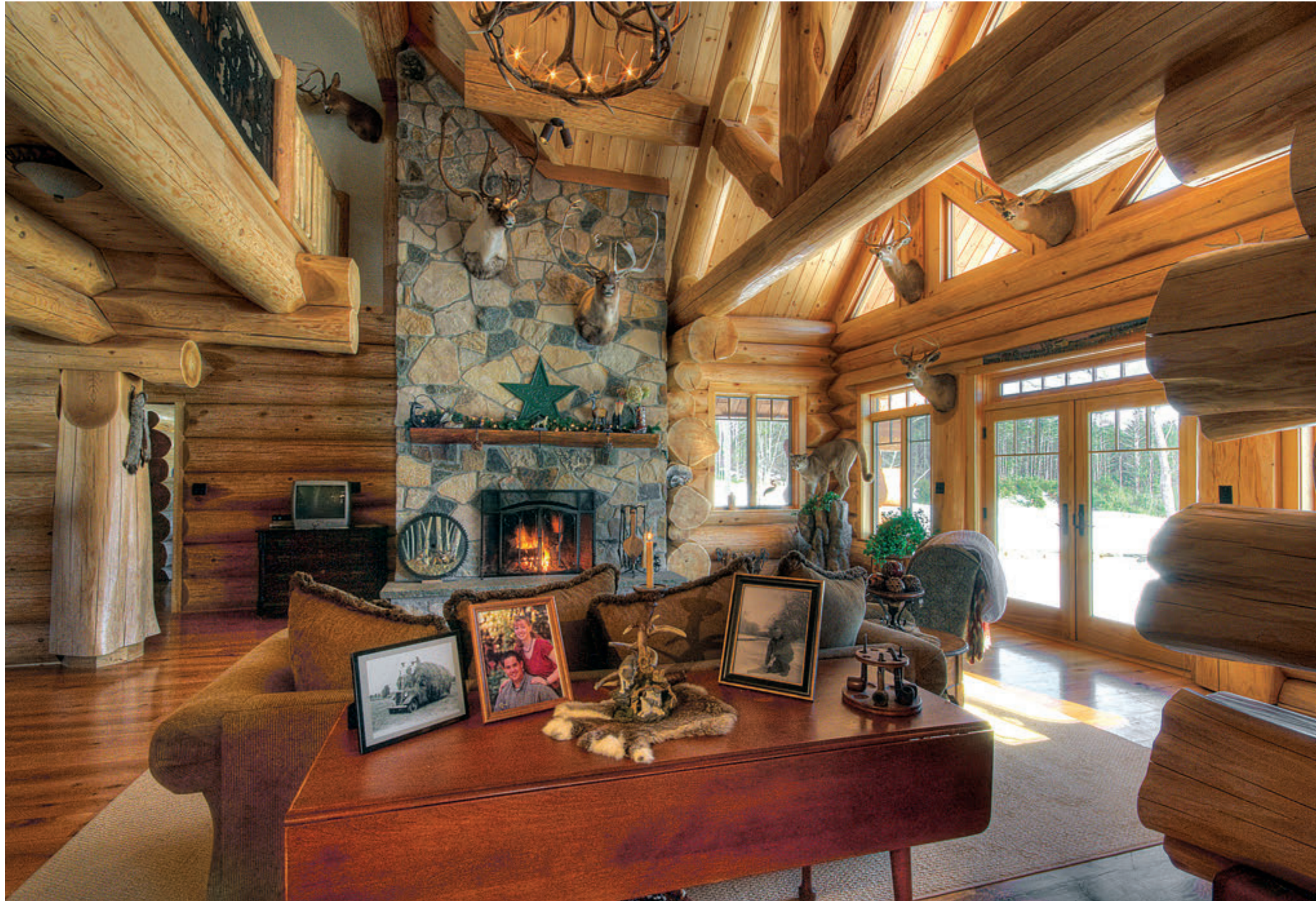
RIGHT: Big logs form the walls, trusses and posts in the great room, where Thomas shows off his trophy mounts. An upholstered sofa and an heirloom drop-leaf table exemplify the old and new furnishings that fill the home. Goshen stone forms the fireplace.
